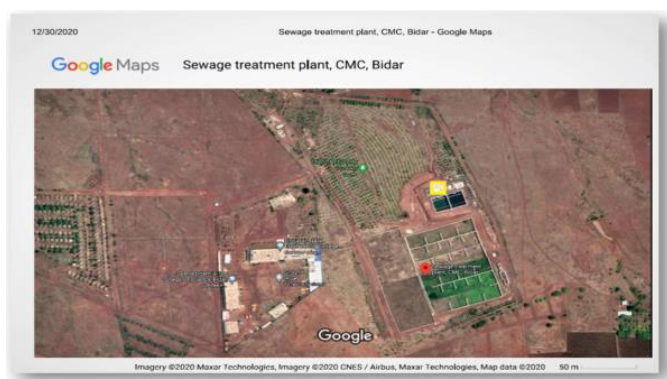
Figure 5. Google Map location of Domestic waste water treatment plant
